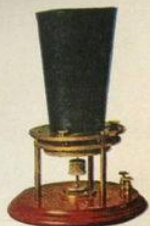
1876 Liquid Telephone. This is Alexander Graham Bell's historic invention which revolutionized communications.
